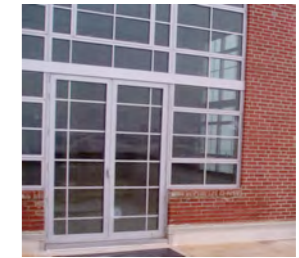
TYPICAL STOREFRONT GLAZING for lower stories
