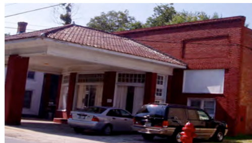
EXISTING GAS STATION CANOPY ON HIGH STREET, CAMBRIDGE
