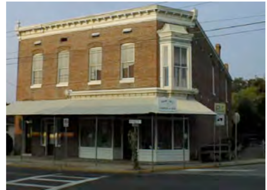
CORNER BUILDING: upper and lower story with cornice at top
