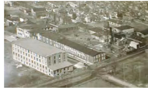
ILLUSTRATION #1: showing Easton Furniture Company circa 1893, with tall multi-floored buildings built into a courtyard configuration, or "work yard" to access and move materials. Also note the simple brick masonry bay system with standard window components to provide adequate lighting and ventilation in interior spaces
