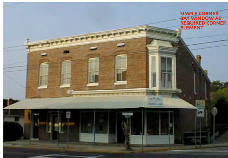
BUILDING CORNER DETAIL: G-4
